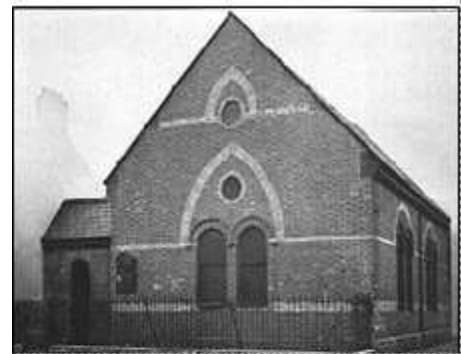
19: Charlotte Street Hall and Schoolhouse
